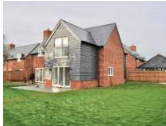
Manor View, Steeple Claydon Completed January 2022
