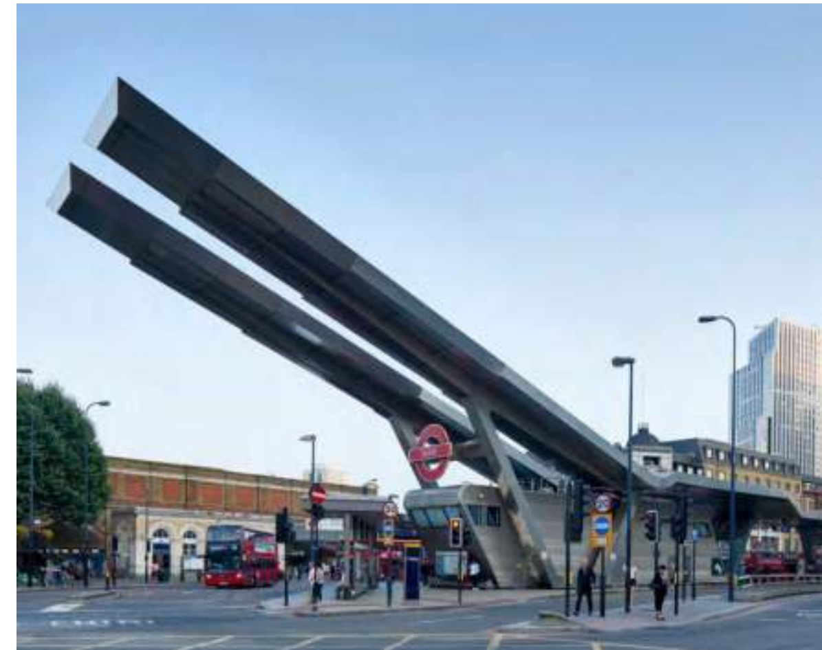
THE BUS STATION WAS DESIGNED BY ARUP ASSOCIATES. IT INCORPORATES TWO CANTILEVERED ARMS THAT CONTAIN 167 SOLAR PANELS.
