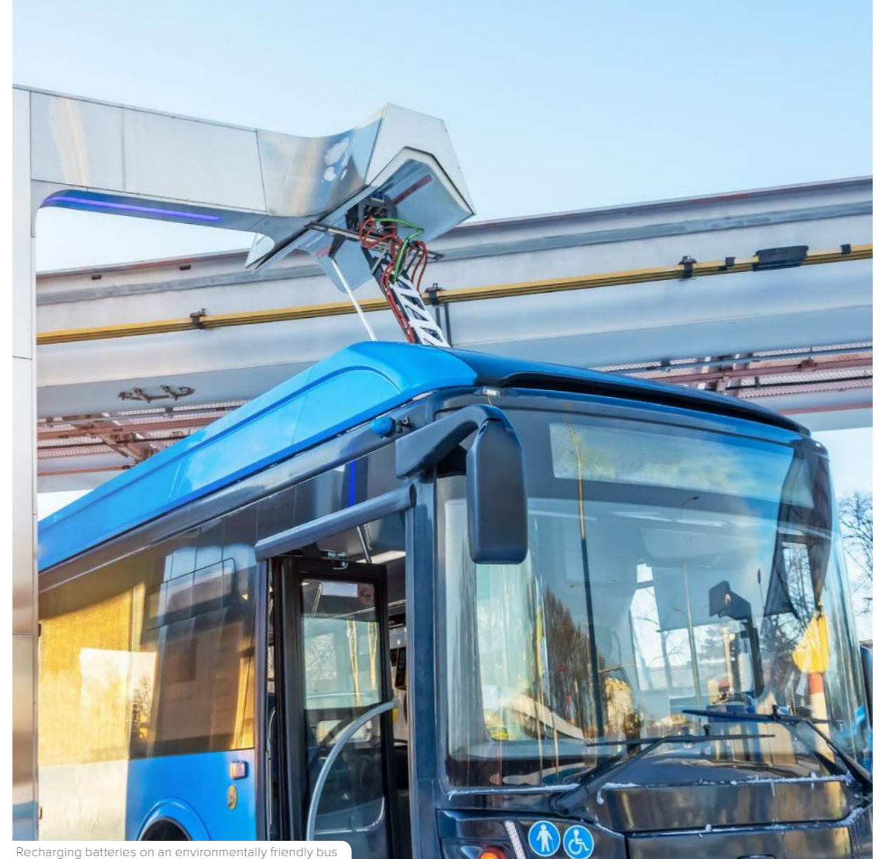
Recharging batteries on an environmentally friendly bus
